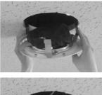
Hook the speaker mounting spring(s) into the mounting hole.
